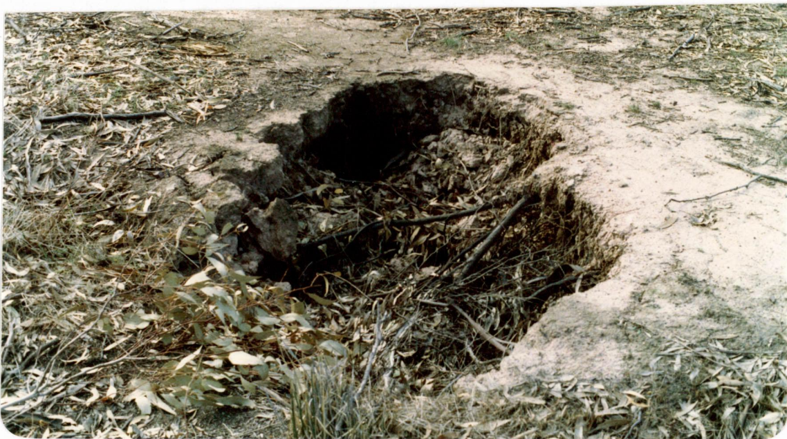
Plate 8 'Sinkhole' (photographed on-site 30/4/'85)
